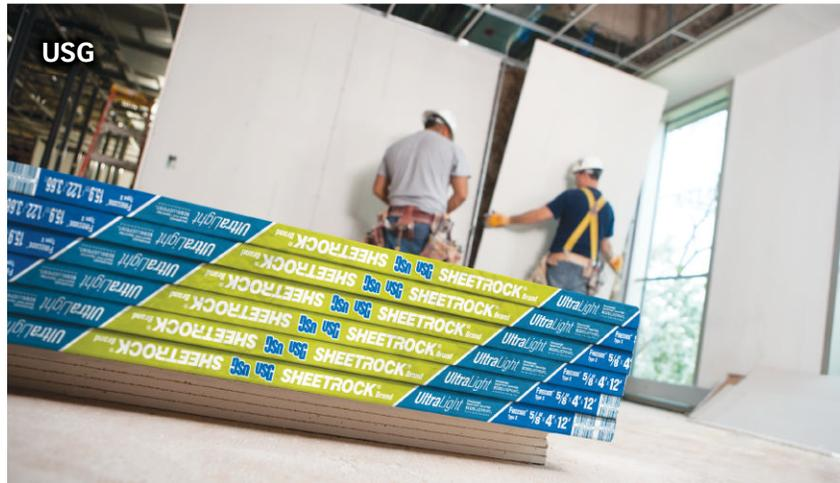
Firefighters: USG's new fire-retardant wallboards are lighter than standard Type X gypsum.
