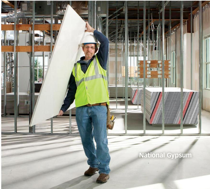
**Lighten Up:** National Gypsum developed 5/8-inch-thick wallboards that slow the spread of fire while weighing 15% less than standard Type X (fire-resistant) gypsum.
